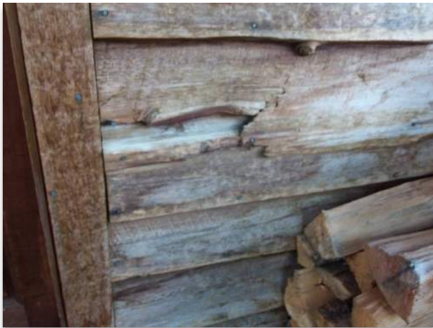
Figure 4. Wood siding in poor condition with firewood stacked against the siding.
