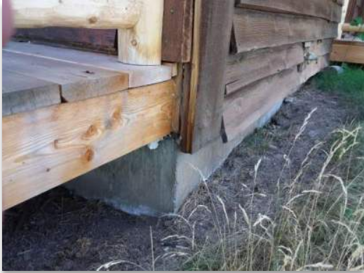
Figure 5. Concrete foundation where siding deteriorated, allowing debris to accumulate and where embers could blow in. The deck should be screened to prevent buildup of flammable materials.
