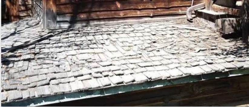
Figure 1. Cedar shake roof in disrepair. Note litter (needles and leaves) collected on the right side of the photo.
